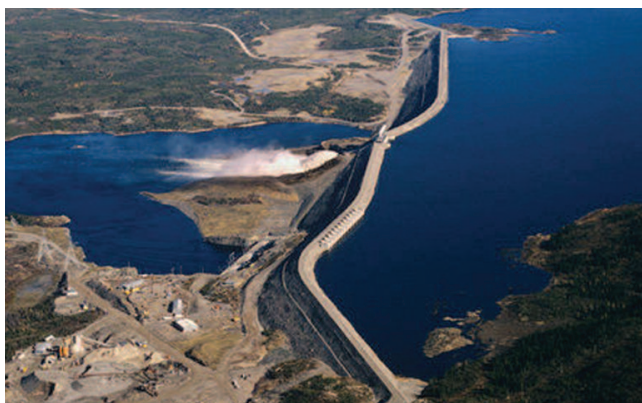
Filling LG 3 reservoir at James Bay induced an earthquake with a magnitude of 3.7
