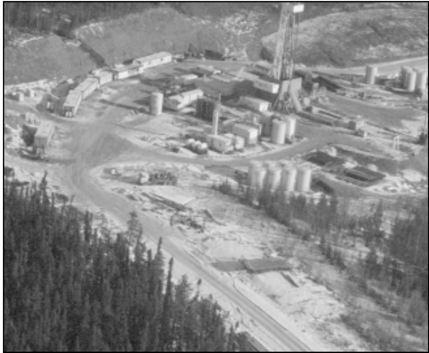
Drilling Operations at the A-5 Location
